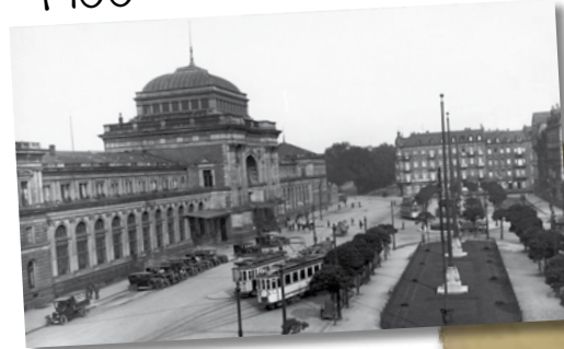
Main Station with entrance hall
